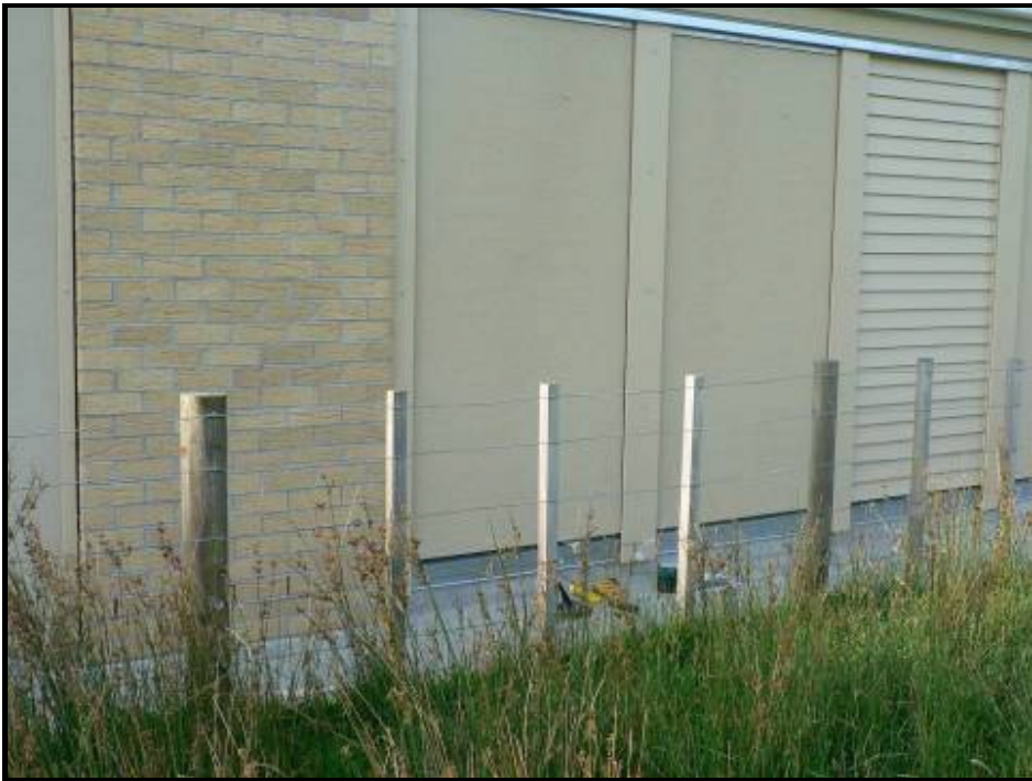
PIC 007 Close-up of typical test panels
