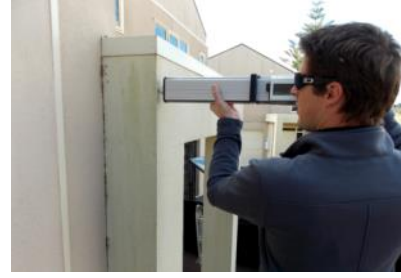
In situ timber assessment
